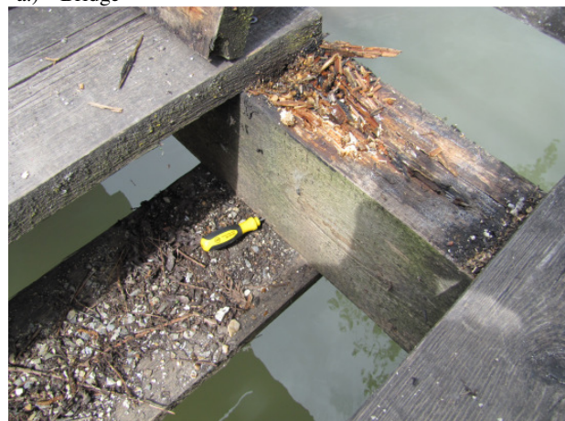
b.) Damage in the range of the joint
